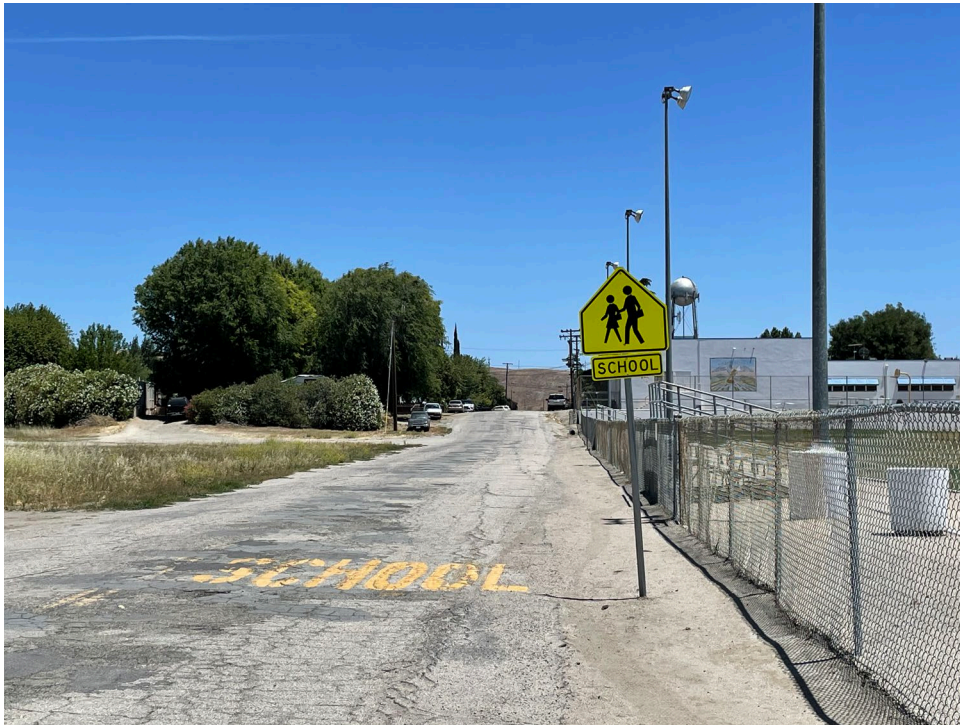
Figure 4 Existing Conditions at Project Site, San Ardo
