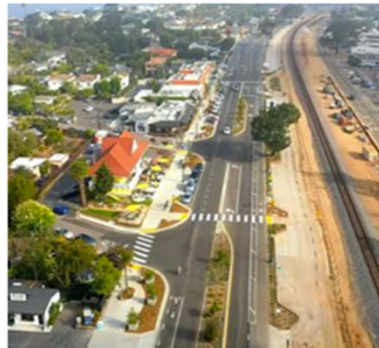
Highway 101 at North Court and Athena St.
