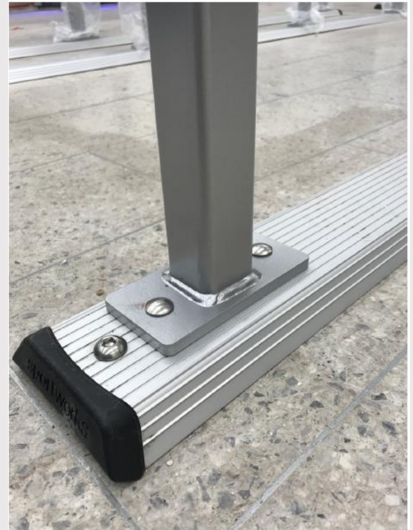
Welded steel flat bar rail-mounted racks anchored to concrete pavers (left); Bolt-on aluminum channel rail-mounted racks anchored to terrazzo floor (right) (Source: APBP Bike Parking Guide – DRAFT)
