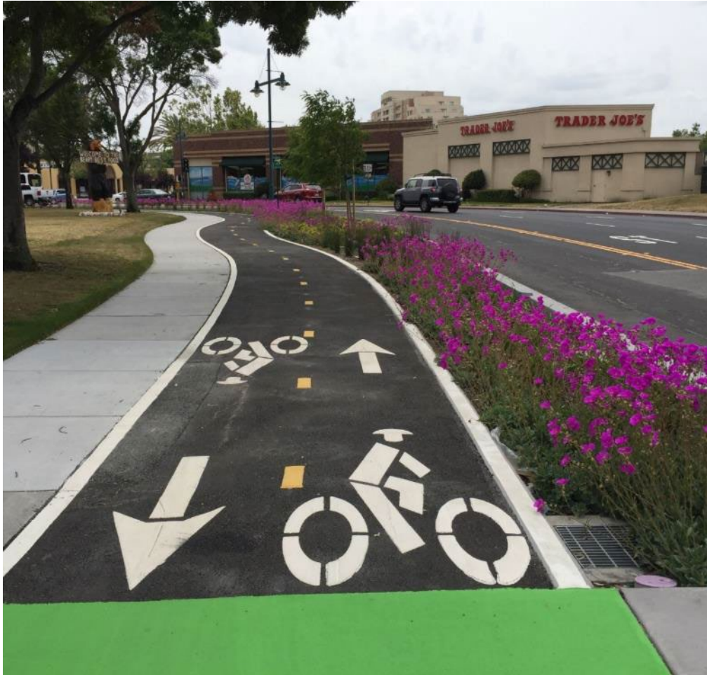
Stormwater cycletrack (Emeryville)
