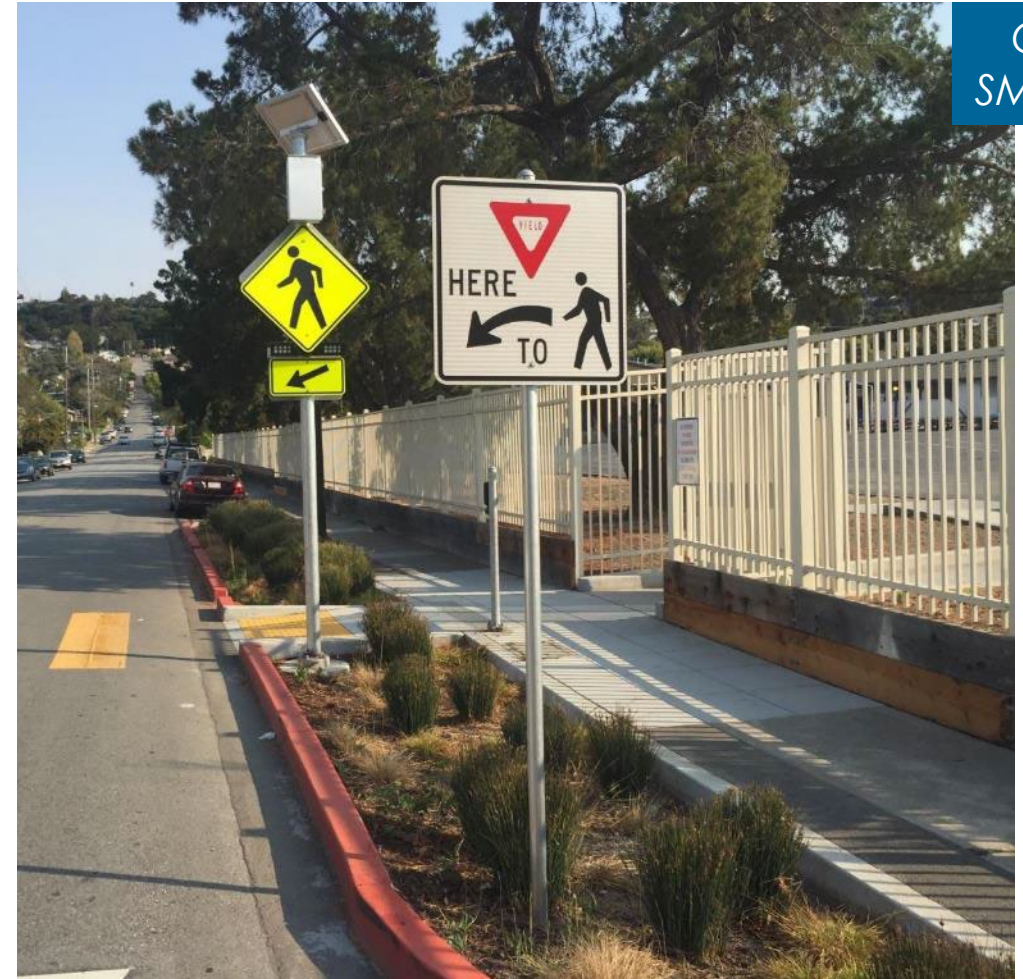
Stormwater curb extension in Safe Routes to School project (San Mateo)
