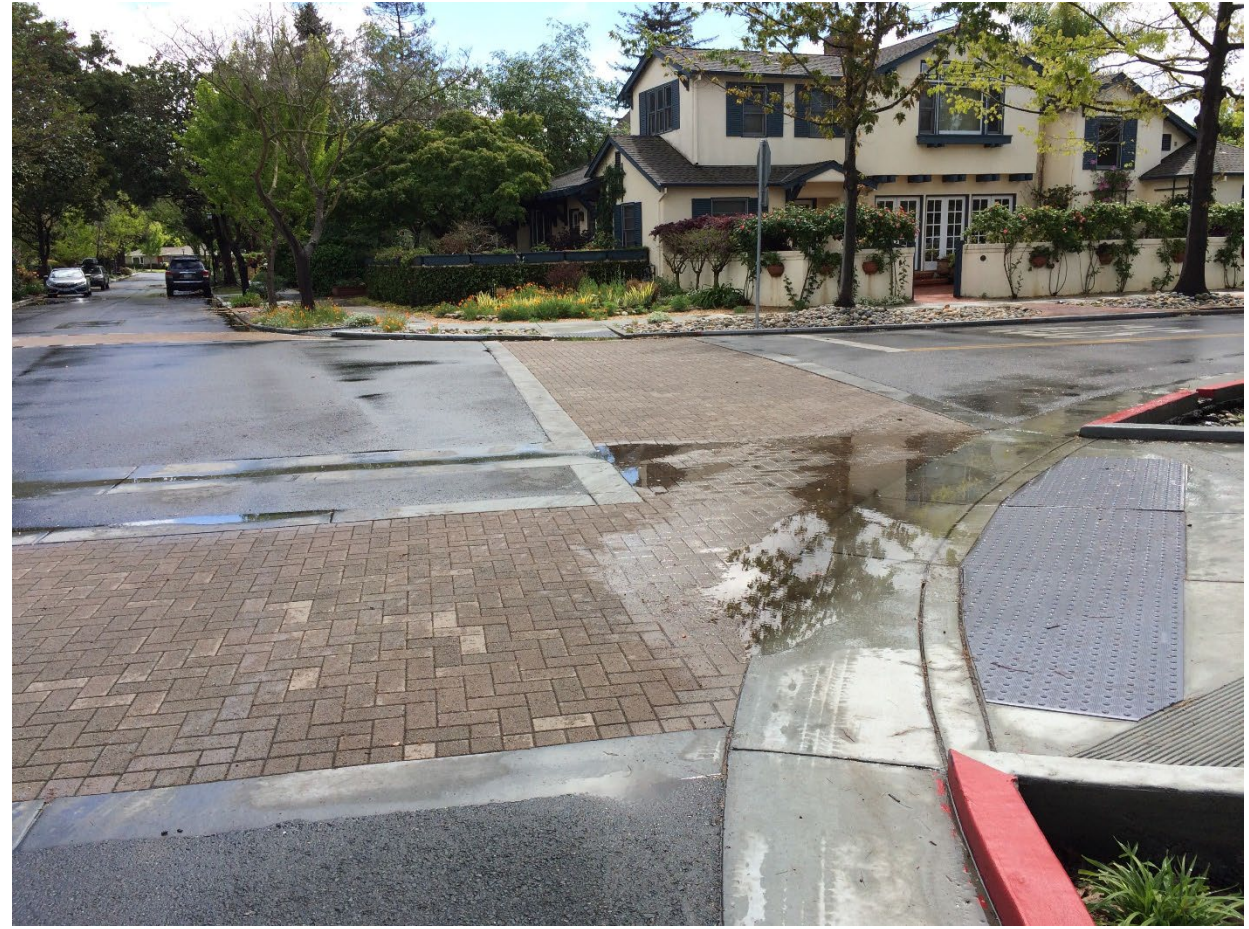
Pervious Paver Crosswalk
