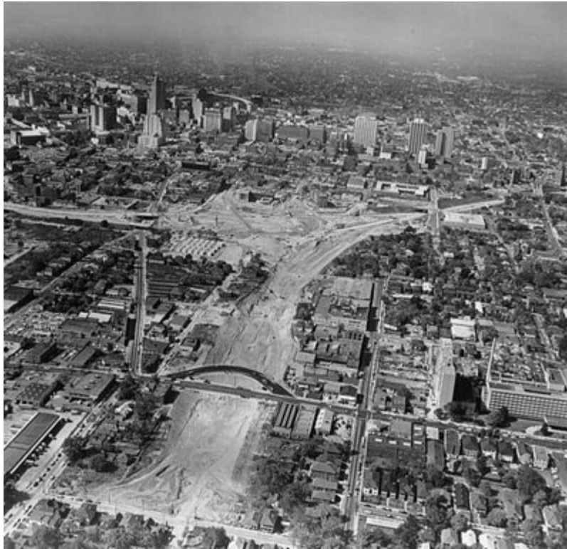
Downtown Atlanta interstate highway construction in 1962 (Source: Darin Givens, twitter.com/atlurbanist/media )
